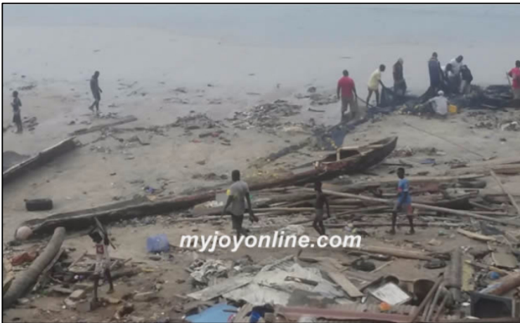
(Property damage of coastal communities in Accra http://www.myjoyonline.com/news/2016/September-5th/accra-fishermen-count-losses-after-tidal-waves-destruction.php )
