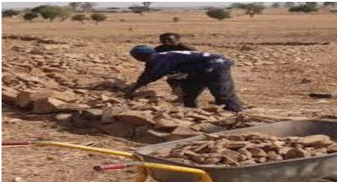
Pic4.2:A 52 year old man in Bawku West gathering stones to construct bunds Farming across slopes (contour faming)
