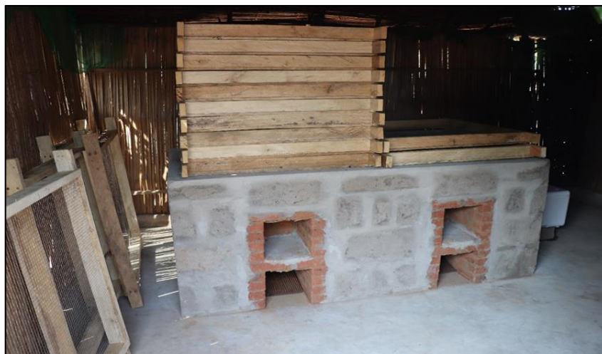
Figure 2. Ahotor Oven with layered fish smoking racks BAP: 2, PAH4: 10.93µg/kg, Price: $400 (GHS 2,500)
