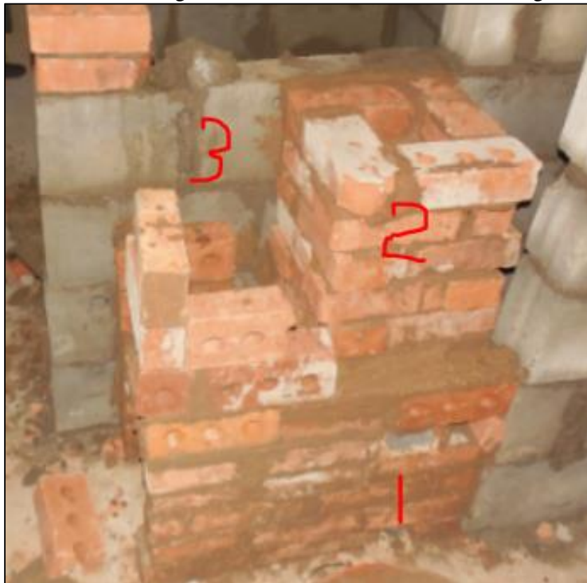
Figure 9 The combustion zone (1) is beneath the brick flame tunnel rising from the right hand end. The hot exhaust gases are then mixed with air in a mixing chamber (3).
