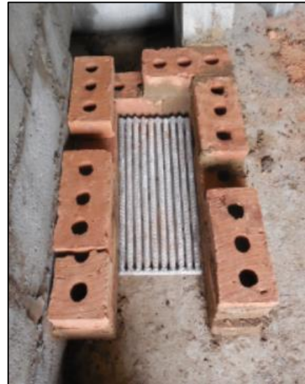
Figure 18 The fire is built upon a grate that sits on the flat floor
