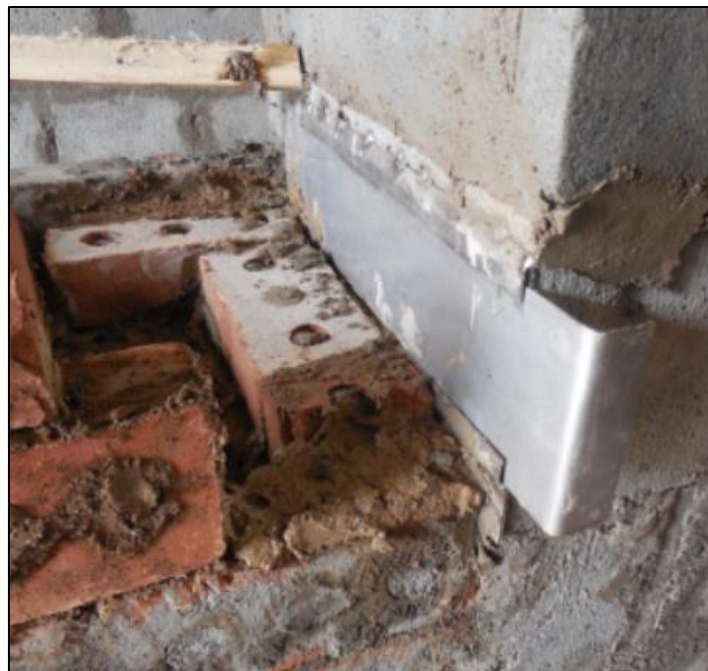
Figure 10 Stainless steel plate slides in a frame to open a vent into the chimney
