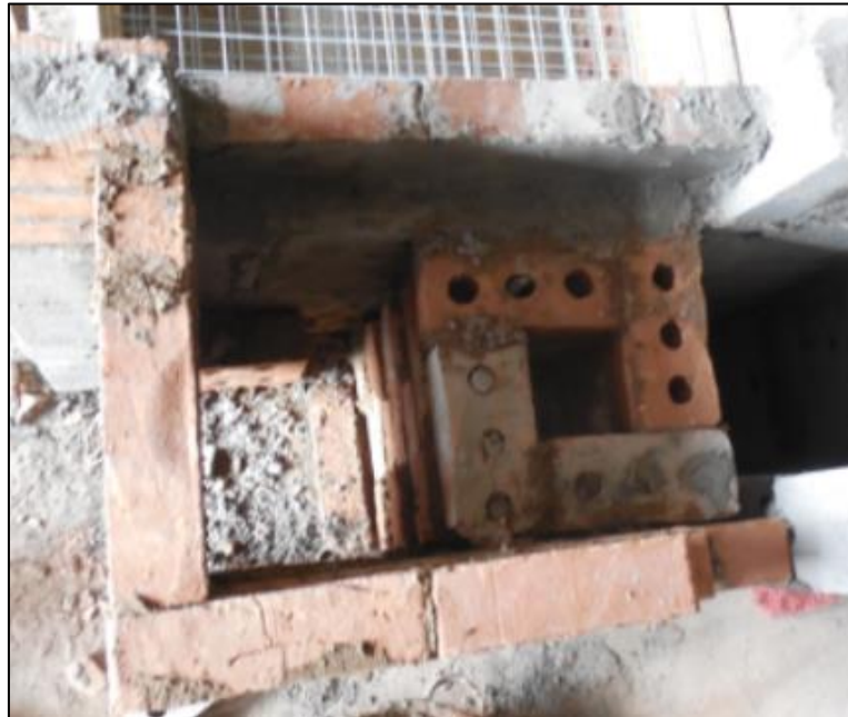
Figure 13 Top of the flame tunnel and drying chamber
