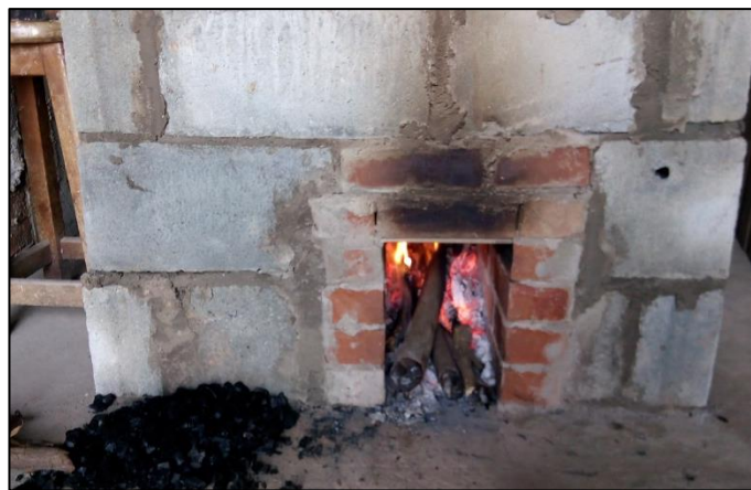
Figure 29 SNV Fish Smoker – Morrison Stove Retrofit View 2
