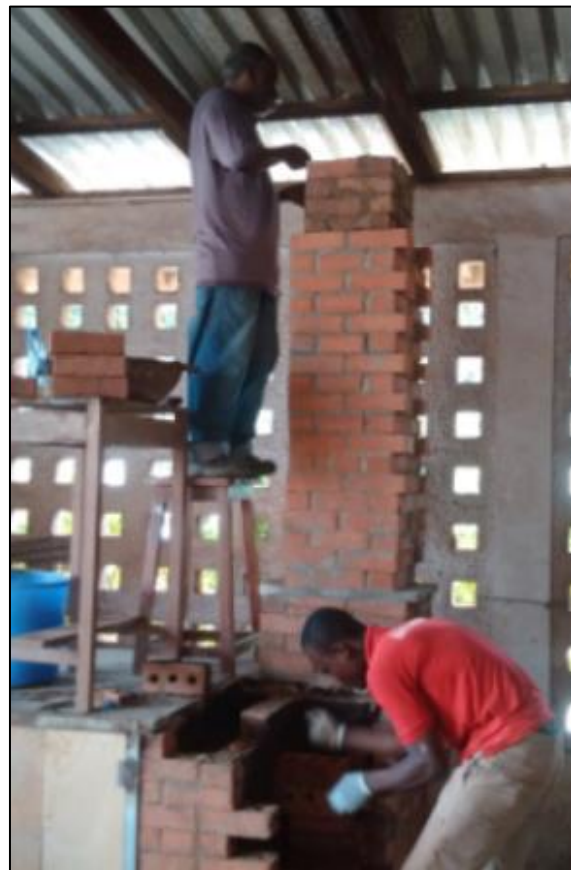
Figure 22 Construction of version 0.4
