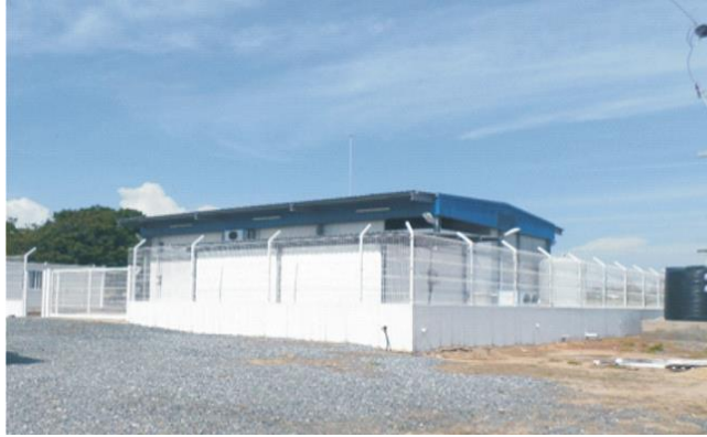
Figure 101. Cold store facility
