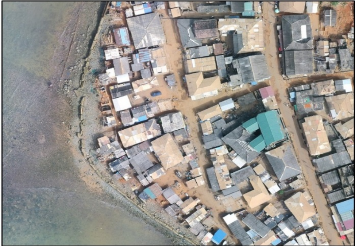
Figure 3: Axim community and collapsing sea defense wall
