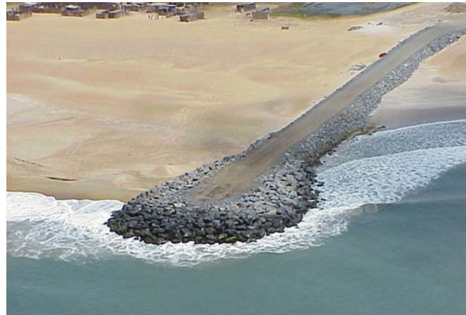
Figure 8: Sea defense structure to mitigate coastal erosion at Keta
