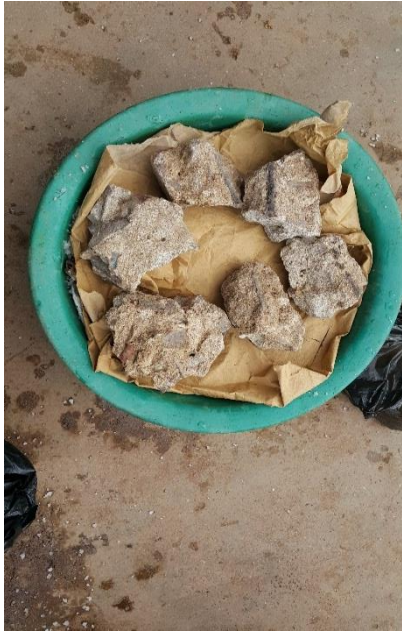
Figure 12 Cover with cement paper and placing stones on top
