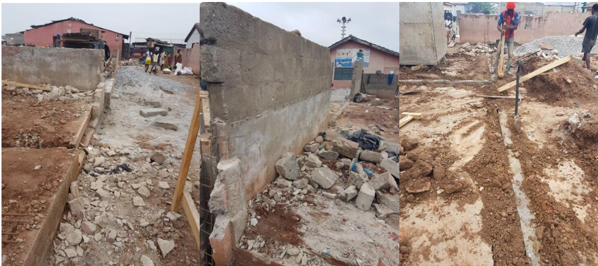
Figure 3 Walls removed as well as column structure being laid
