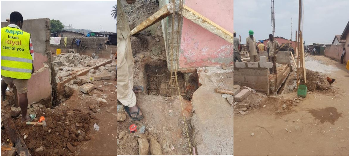
Figure 2 New structure being laid
