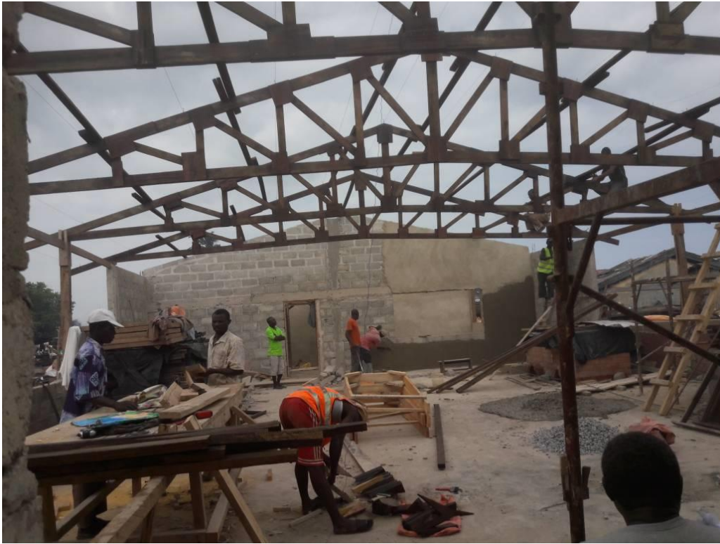
Figure 5 Inside Structure on September 9, 2017
