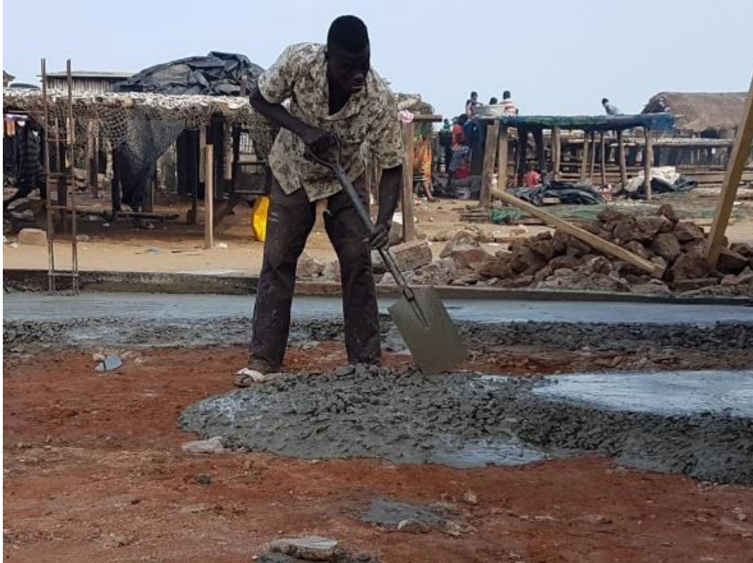
Figure 4 Flooring being laid
