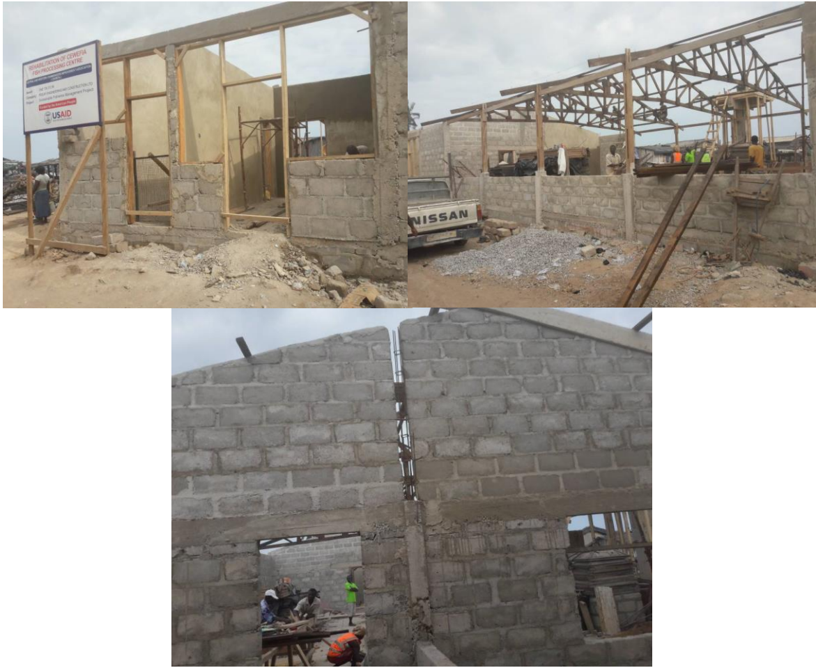
Figure 7 Structure on September 18, 2017
