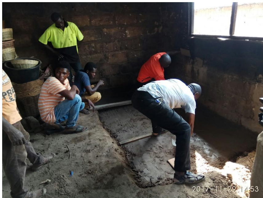
Figure 5 Participants constructing a platform about 6 inch into the ground
