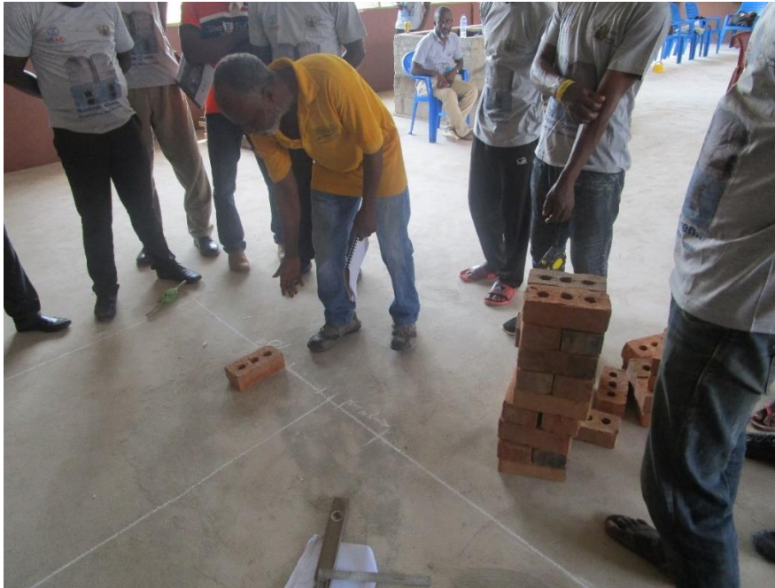
Figure 4 Demonstrator illustrating how to lay the bricks and blocks on the demarcated lines to participants
