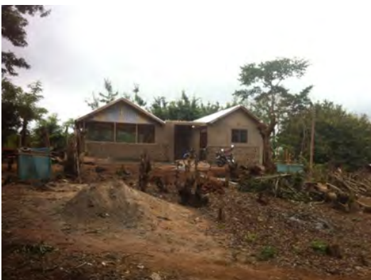
Nearly complete Cashew Facility during construction.
