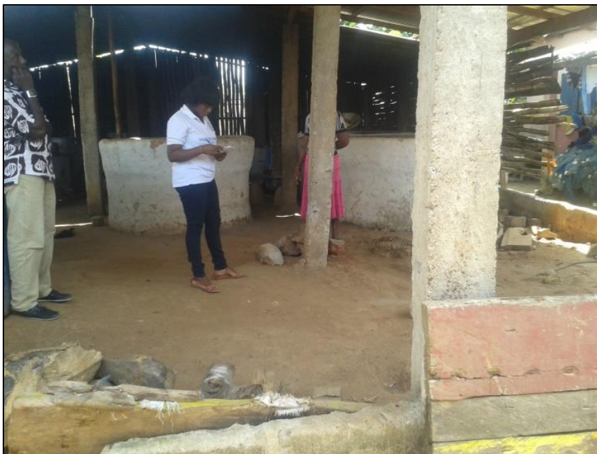
Figure 12. Site inspection for the Daasgift Quality Foundation Model Kitchen
