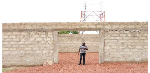
A 200-MT capacity warehouse under construction by the Samakuse Farmers Group
