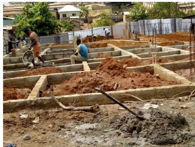
Men at washroom construction site in Techiman
