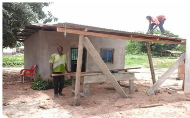
New office under construction by OB Bunbas for business operations
