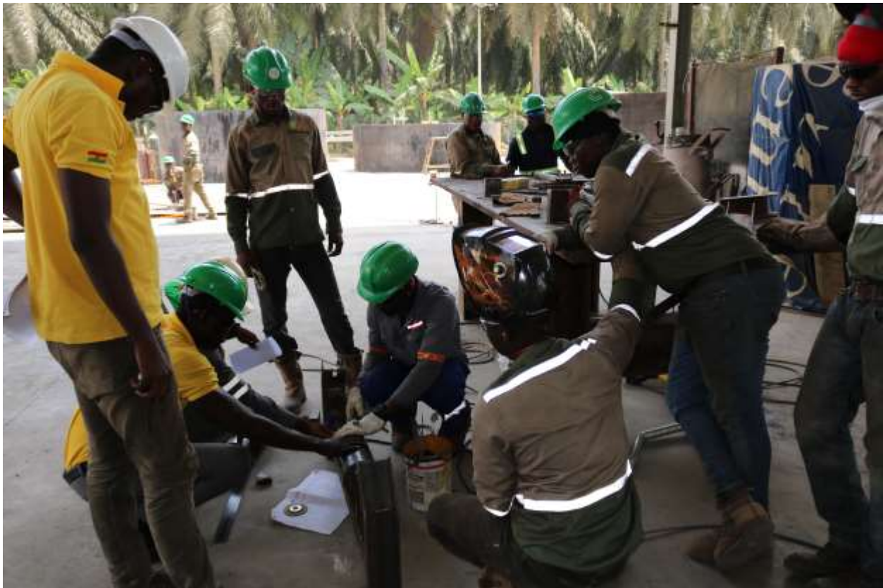
Welders receiving on the job training at Wayoe Engineering and Construction Limited
