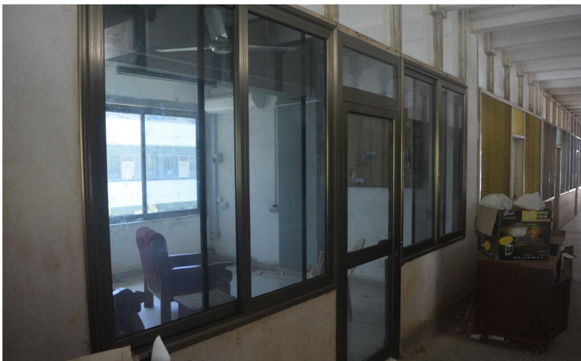
Offices being refurbished for DFAS lecturers to enhance teaching and learning
